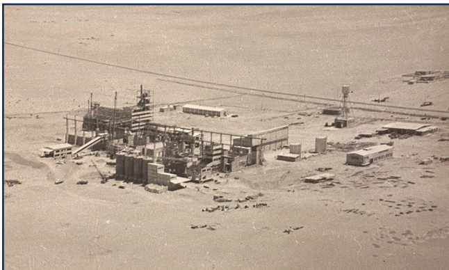
13 An Image Taken in 1956 Documenting the Construction of Al-Yamamah Cement Company's Factory.
