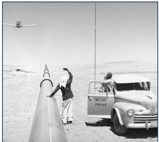
08 Aided by an aerial survey, a work crew inspects the Tapline oil pipeline in 1951
